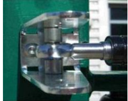
Figure #2 Post Bracket with Spacers and Gate Closer attached.
