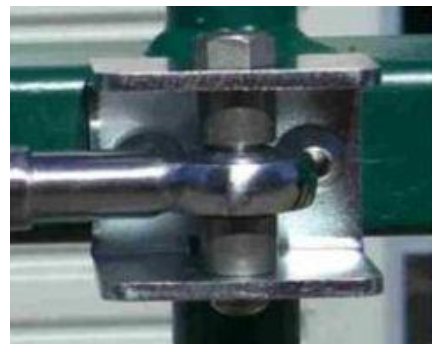
Gate Bracket with Spacers and Gate Closer attached.
